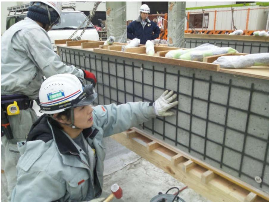
Figure 4-7: CFRP Grid is fixed to two sides of RC beam 2 and 3
