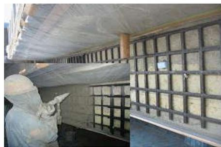
b) Shear reinforcement
