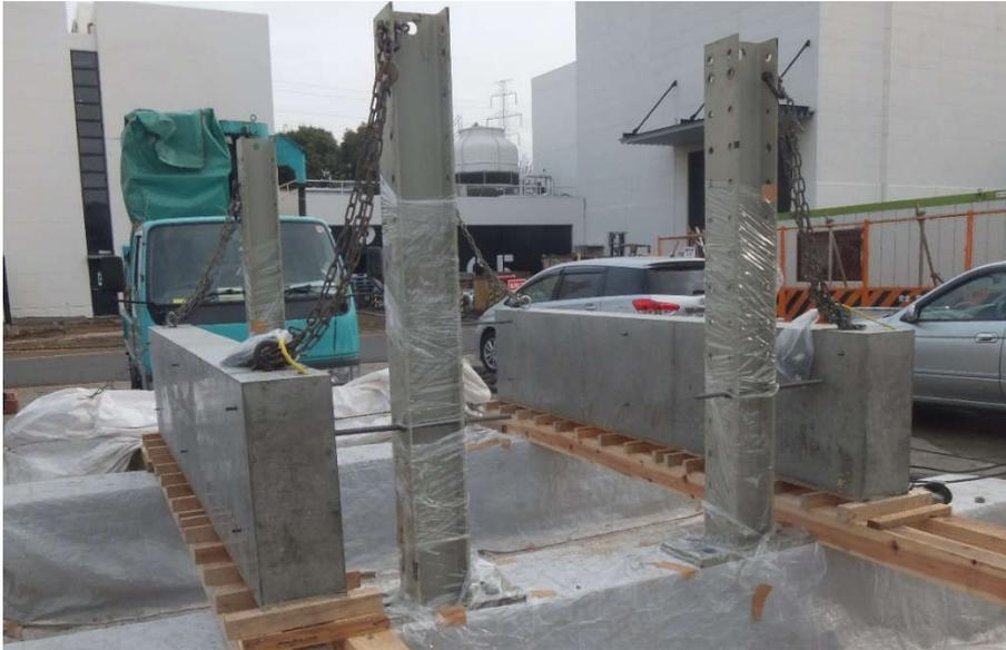
Figure 4-6: Concrete beam after demolding
