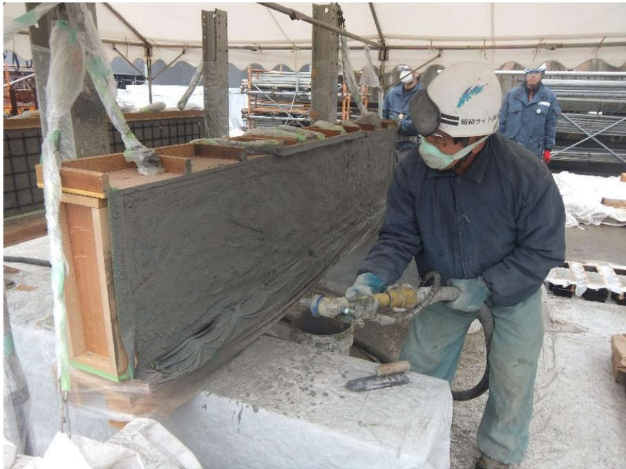
Figure 4-8: Spraying the mortar to RC beam 2 and 3
