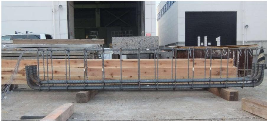
Figure 4-3: Reinforcing bars and stirrups
