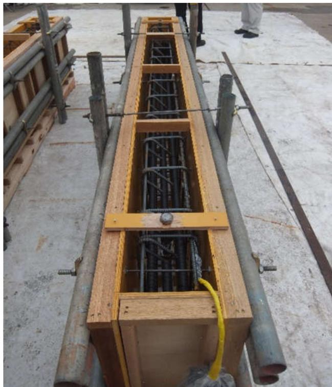
Figure 4-5: Reinforcing bars placed in wooden formwork before casting concrete
