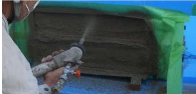
Figure 3-6: Spraying mortar
