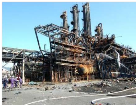
Figure 1.3 Vinyl chloride monomer facility
