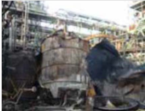
Figure 1.5 Acrylic acid manufacturing facility
