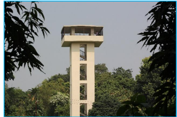
Figure 6.28 Watch tower (EL) Taken by the author, November 2015
