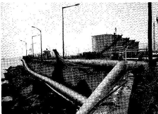
Fig.12 Piping Falling from the Embankment Wall
